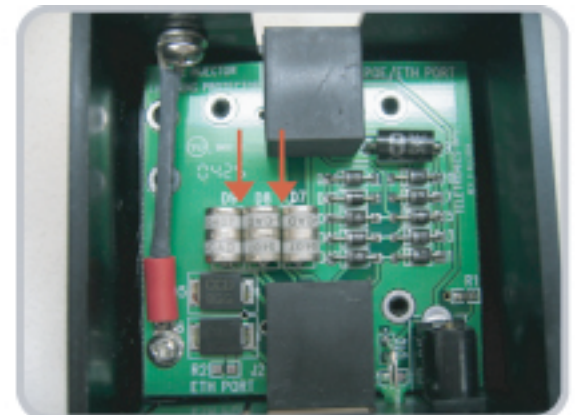
Figure 3: These 3 components do not have sufficient clearance.
